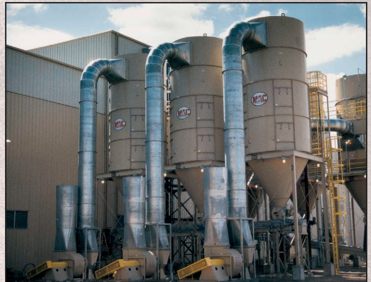
ABOVE Refuse-derived fuel installation with high-entry inlets and wide bag spacing designed for lightweight material.
